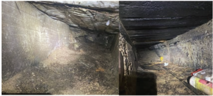
Tunnel No. 1 from garage to basement kitchen. Partially collapsed tunnel from garage west to basement. Notice the rail on the floor in the photo on the right of the approximately 3x3-foot tunnel. (photo courtesy of Harbor Springs Museum)
