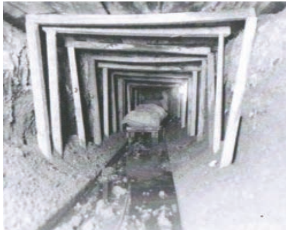
Tunnel No. 1 from garage to basement kitchen. Partially collapsed tunnel from garage west to basement. Notice the rail on the floor in the photo on the right of the approximately 3x3-foot tunnel. (photo courtesy of Harbor Springs Museum)
