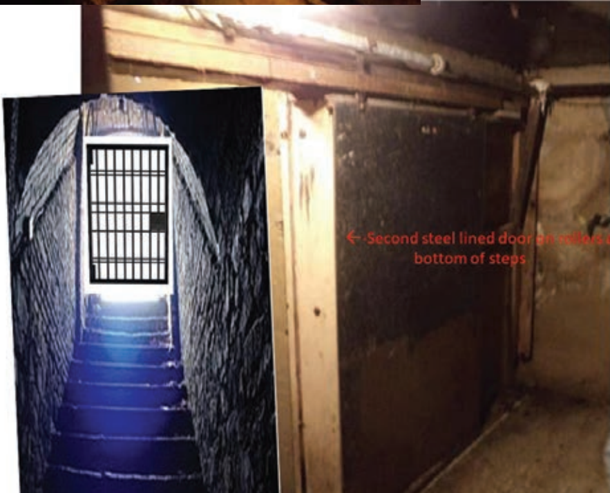
Second steel-lined door on rollers at the bottom of the steps.
