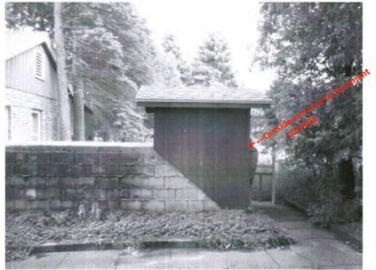
Outside entrance to basement lounge.
