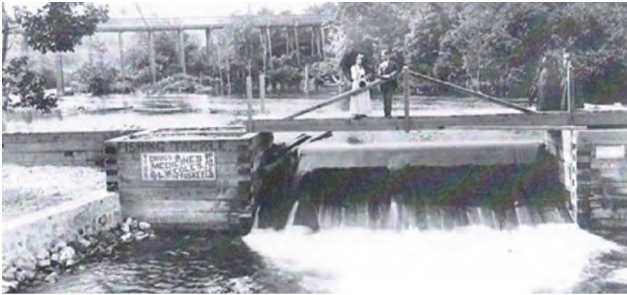
Lake Street Dam
