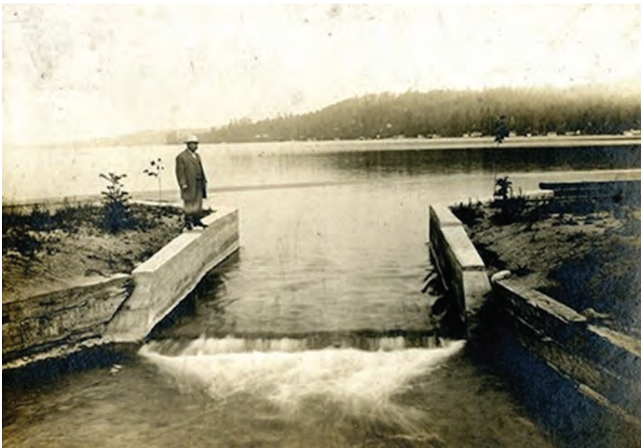
Bear River Dam at Walloon Lake
