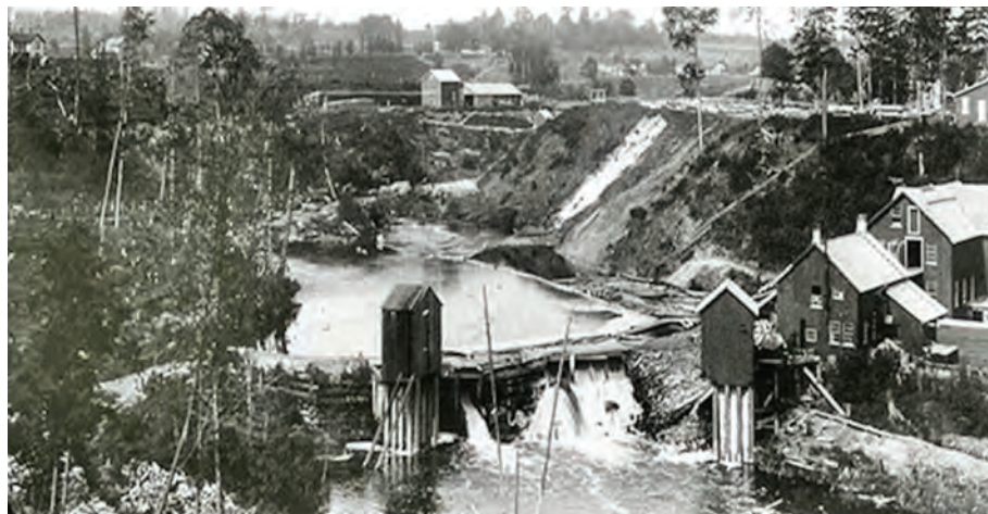
Gardner-Hankey dam built in 1879 just upstream (south) of Shaw & McMillan Dam
