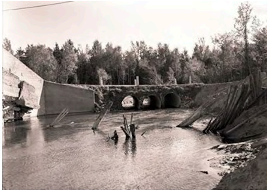
Woodland Road culverts 1952-1967
