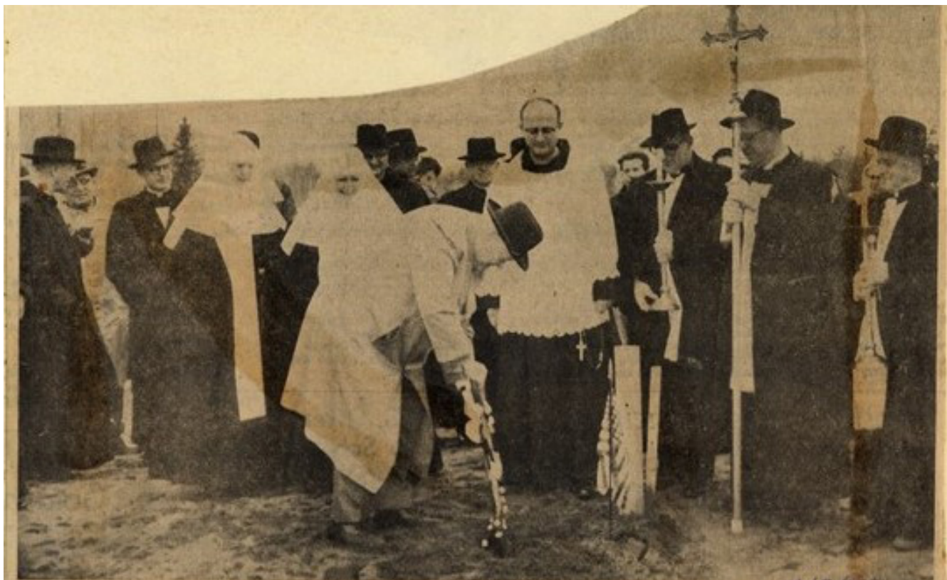
OFFICIAL GROUNDBREAKING took place yesterday afternoon at Conway for the new $550,000 Sacramentine monastery and retreat house, attracting several priests and church members in the area. Shown above is Henry Galster, co-chairman of the fund drive from Petoskey, turning over a shovel of dirt. Others taking part in the ceremonies included Rev. Fr. Laurin Buzinski, pastor of St. Francis in the center who delivered the address on behalf of Bishop Allen J. Babcock of Grand Rapids and Mother Superior Mary Augustine of the Sacramentine Sister at the left is Assistant Mary of the Incarnation. Rev. Fr. John Sheehy, third from left, of Cheboygan, delivered the address of dedication. On the right are acolytes Fr. Kloniwicz, Elmira, and Fr. Decker of Indian River and cross bearer Fr. Max Ostrowski of
