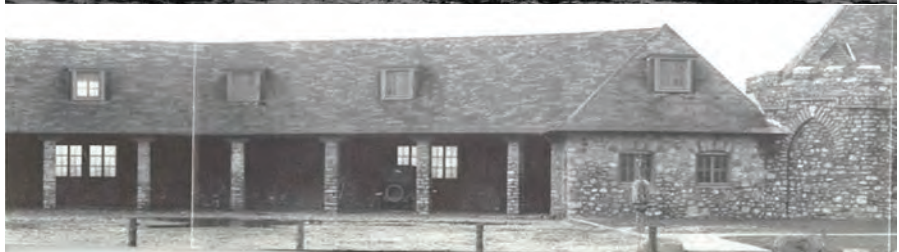
The Carriage Hall was originally an open air structure that housed buggies and automobiles during the days of Loeb Farms.
