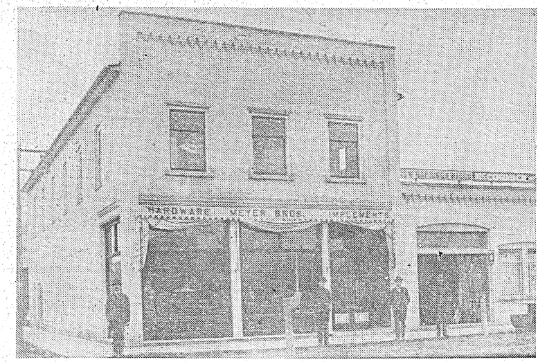
1903 . . . Exterior of Boyne Falls Store
